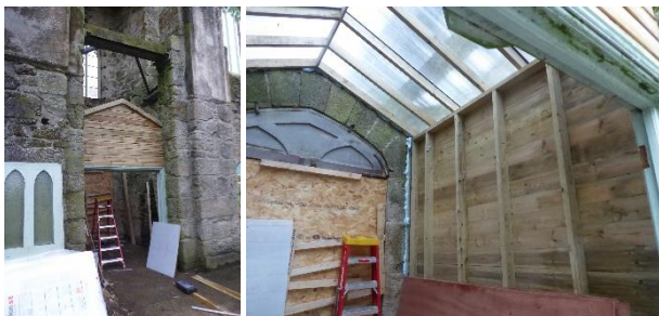
Construction of the 'inner vestibule'
